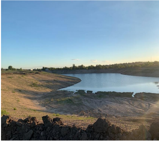
Walker Pit Reservoir
