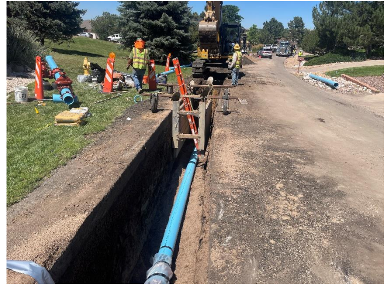
Hillside Way Water Replacement 2023
