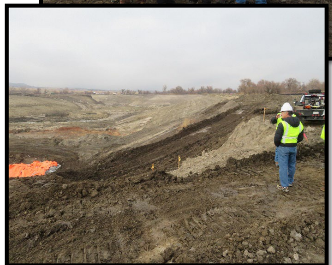
Pinery Board and Efficiency Task Force tour of construction December 2023
