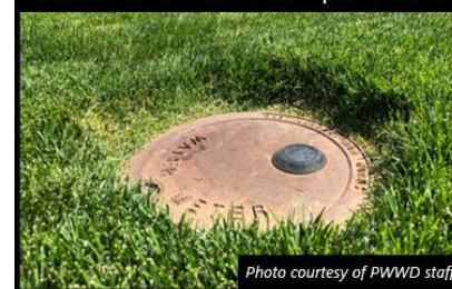
Well maintained meter pit access
