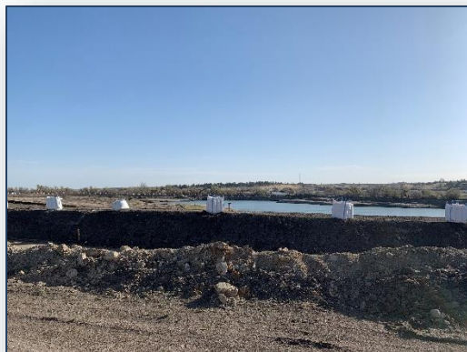
Walker Pit Construction. Photo Credit: David M.
