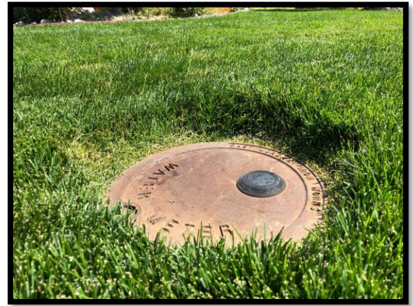
An example of a well-maintained meter pit.
