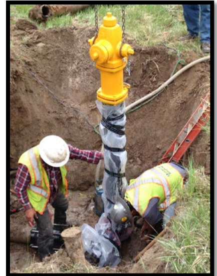
Fire hydrant replacement
